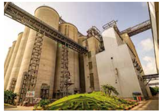
CP Vietnam's Hai Duong feed mill showcases state-of-the-art, fully automated technology and a robotic pallet stacking system. With capacity of 720,000 tonnes/year, it serves customers in North Vietnam.
